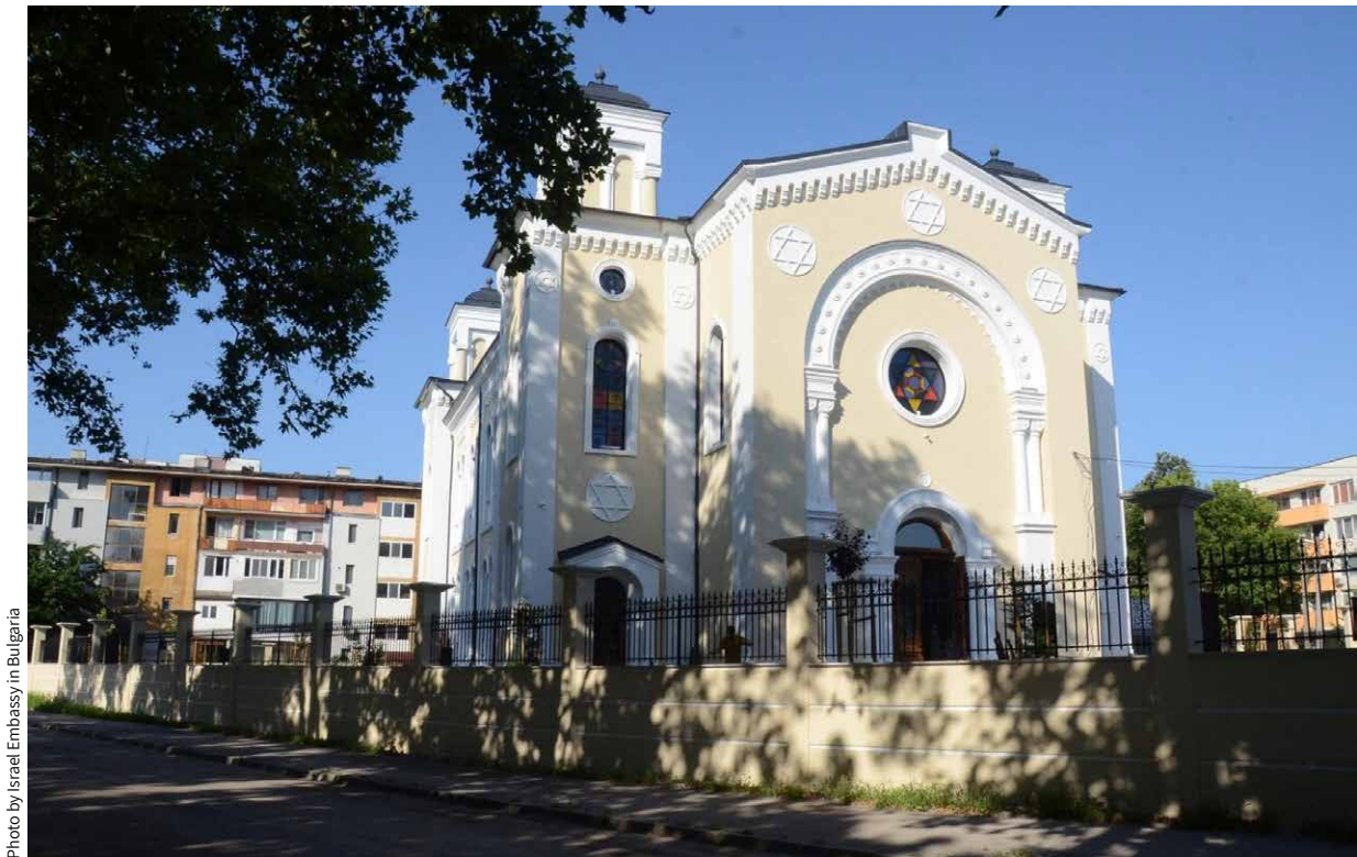
The Vidin Synagogue Before and After Renovation
